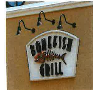
Gooseneck light fixtures angled and shielded so that the bulbs are not exposed.
