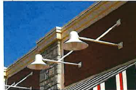
Gooseneck light fixtures that are not angled downward leave the bulbs exposed and create glare.
